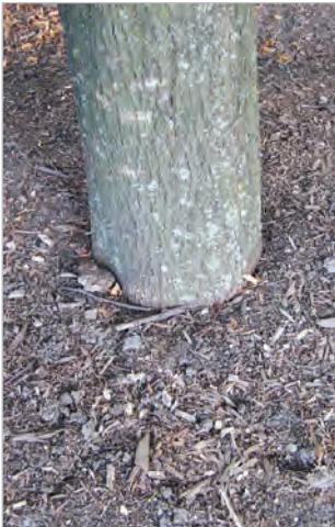
Soil piled up to the base of the tree; root flare is buried.
