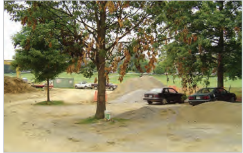
Top soil removed and subsoil compacted around the bases of the tree. Photo: Eric Wiseman, Virginia Tech
