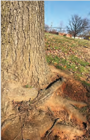
Girdling roots cause constriction along the base of a tree. Photo: VDOF
