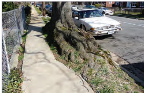
Constricted roots will find various places to grow including under paved infrastructure. Photo: VDOF
